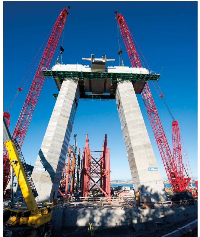
Figure 7. Lower cross beam center box placement.
