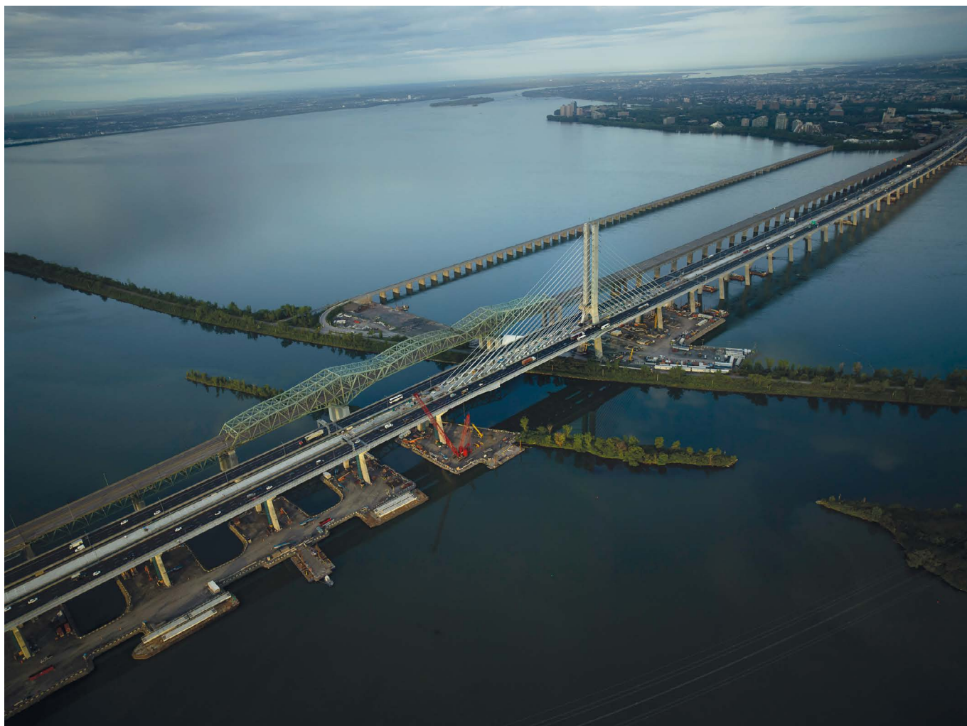
Figure 20. The new Samuel De Champlain Bridge featuring the cable-stayed bridge span at completion.
