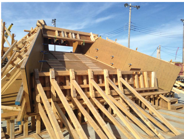
Figure 9. Bow tie formwork
