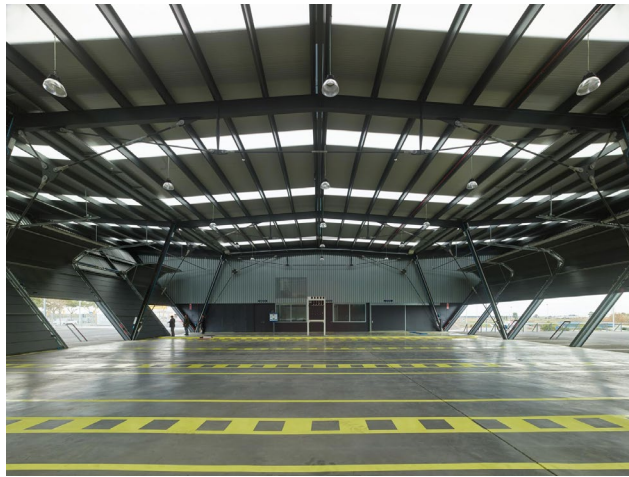
Figure 11. Photo of the Skelsion portal frames © Roland Halbe.
