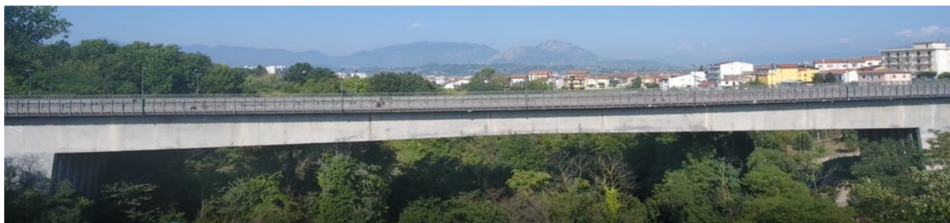
Figure 1. Current lateral view of San Nicola Bridge.
