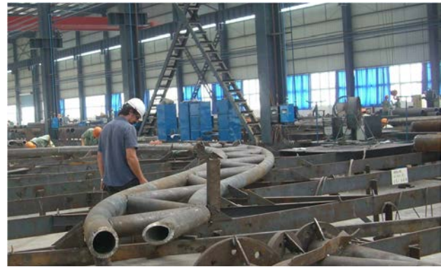
Figura 35. Celosía vertical en construcción Figure 35. Vertical curved truss system under construction
