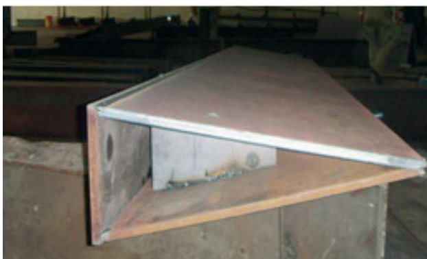
Figura 19. Viga triangular en construcción en taller (tumbada) Figure 19. Triangular beam under manufacture at the workshop (turned)
