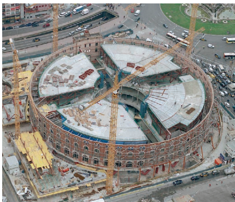
Figura 41. Vista general con el nivel 4 ya hormigonado Figure 41. General view after level-4 concrete was cast
