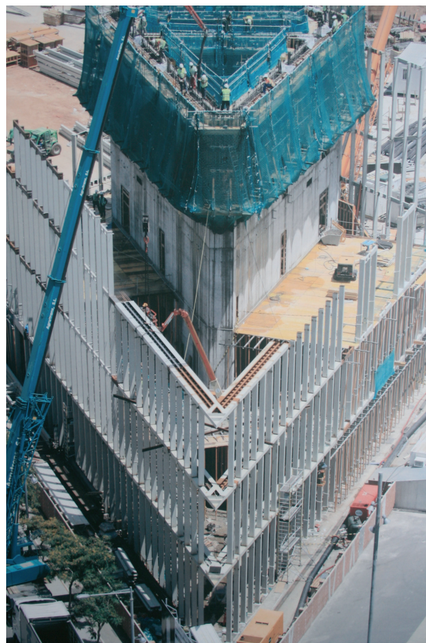
Figura 7. Avance de fachada y núcleo Figure 7. Concrete core and steel facade under construction
