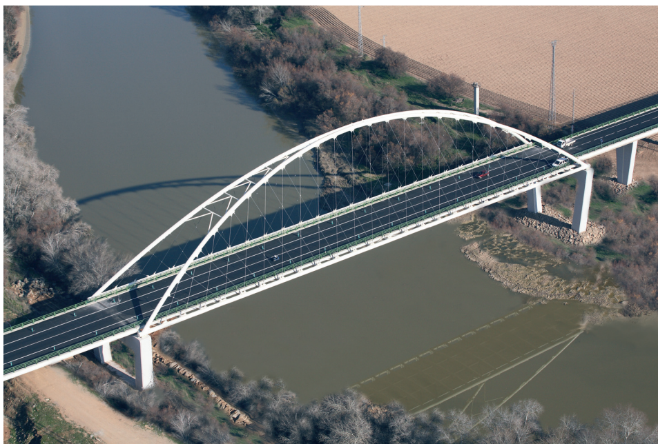
Figura 31. Vista aérea del Puente Arco sobre el río Guadalquivir Figure 31. Bird's eye view of the Arch Bridge over River Guadalquivir
