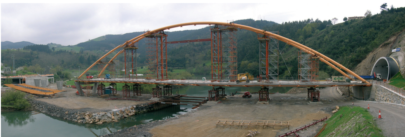
Figura 28. Vista del arco y tablero apeados Figura 28. View of the arch and deck while shored
