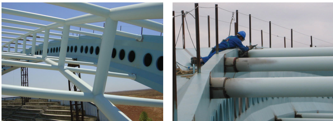
Figura 39. Uniones terminadas de tubos y cajón con teja y contra-teja. Figure 39. Finished joints of the tubes and caisson with dowels and counterdowels.
