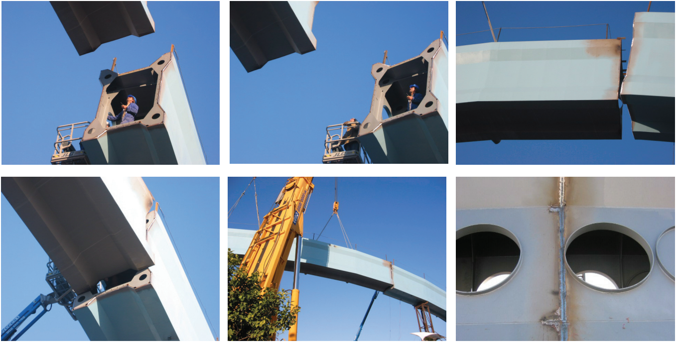
Figuras 37. Uniones a tope de los cajones. Figure 37. Butt joints of the caissons.
