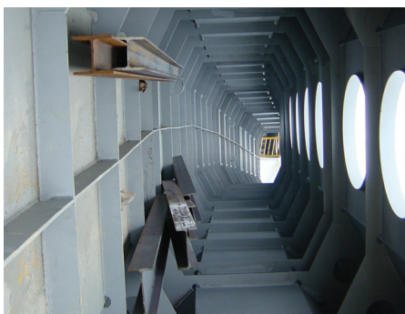
Figura 43. Aspecto del pasillo interior reforzado con los rigidizadores. Figure 43. Appearance of the interior corridor with the reinforcement of the stiffeners.
