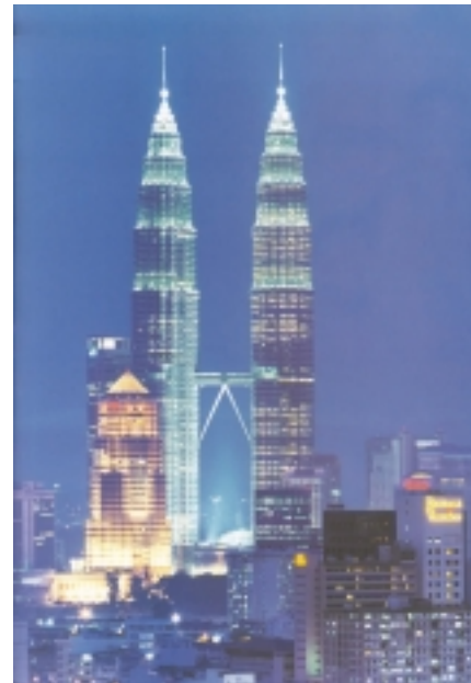
Figura 5. Torres Petronas, Kuala Lumpur.
