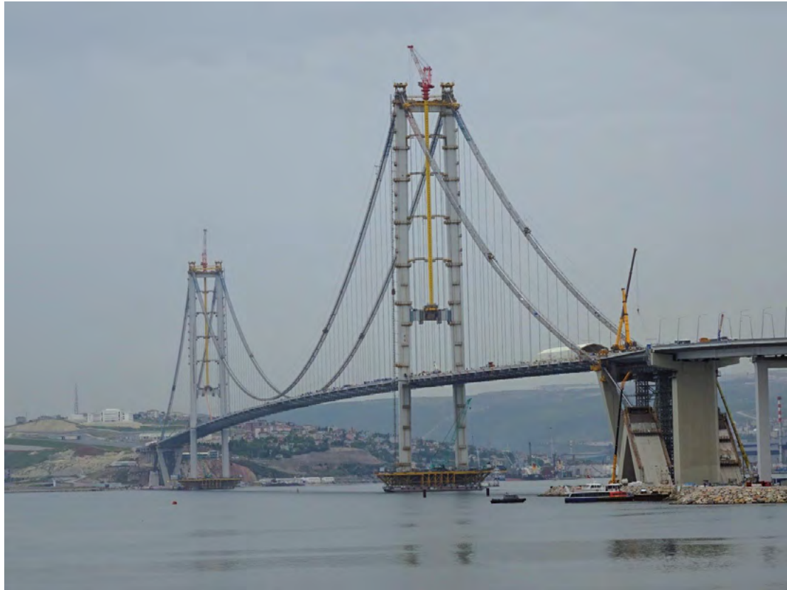
Figure 1. Osmangazi Bridge, Turkey, 2016; 1550 m main span.
